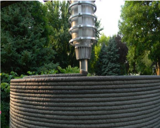
Figure 3: A 3D printing of a house [6]
